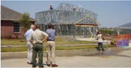
Project managers oversee framing construction.
